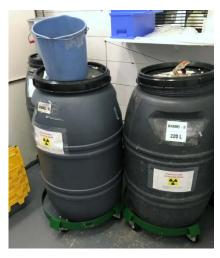
**Photo 8:** Liquid effluent collection drums in Zone 3 with new labels posted after inspection
